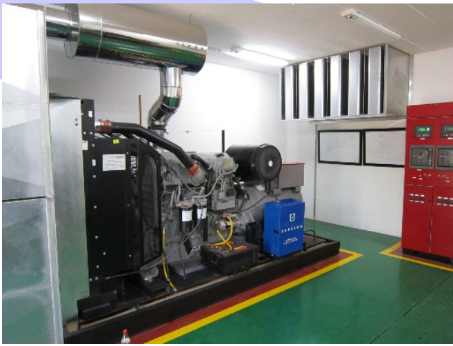
Netcare Montana Standby Generator installation. 2x 500kVA Prime rated sets synchronised to operate at a total supply of 1MVA
